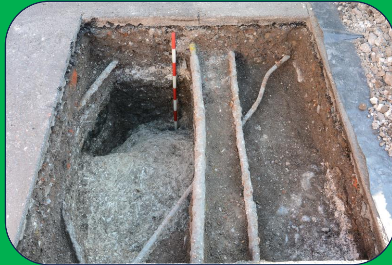
Trial Pit Four after excavation
